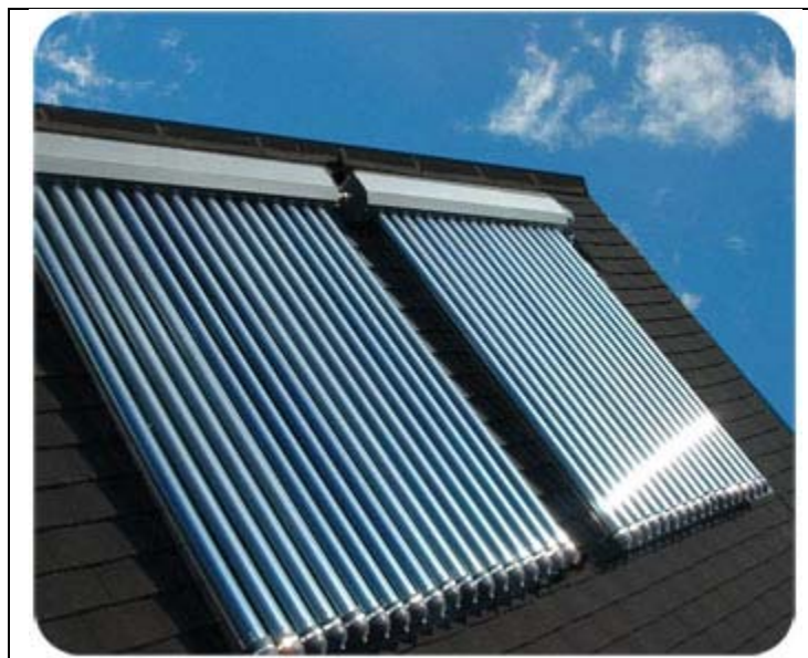
Figure 1: Solar Thermal Collector
